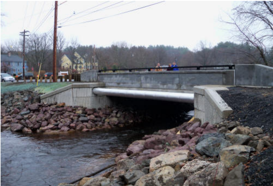
The Selectmen and Town Manager Richard Reed attended a ribbon cutting ceremony for the opening of the Page Road Bridge on November 24, 2009
